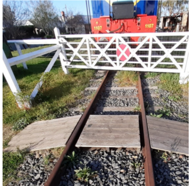
Fig. 4 A typical walk way of planks on the Bellarine Peninsula Railway in Victoria.
