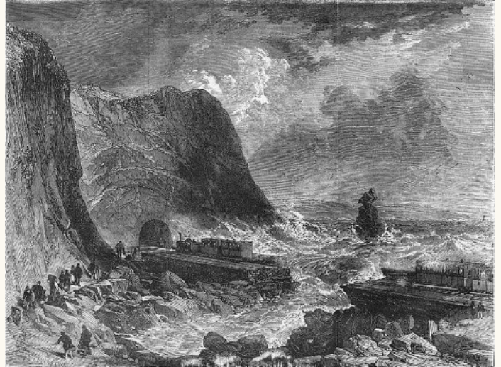
Fig. 1 The drawing that started it all – the 1855 collapse of the Dawlish (England) sea wall.
